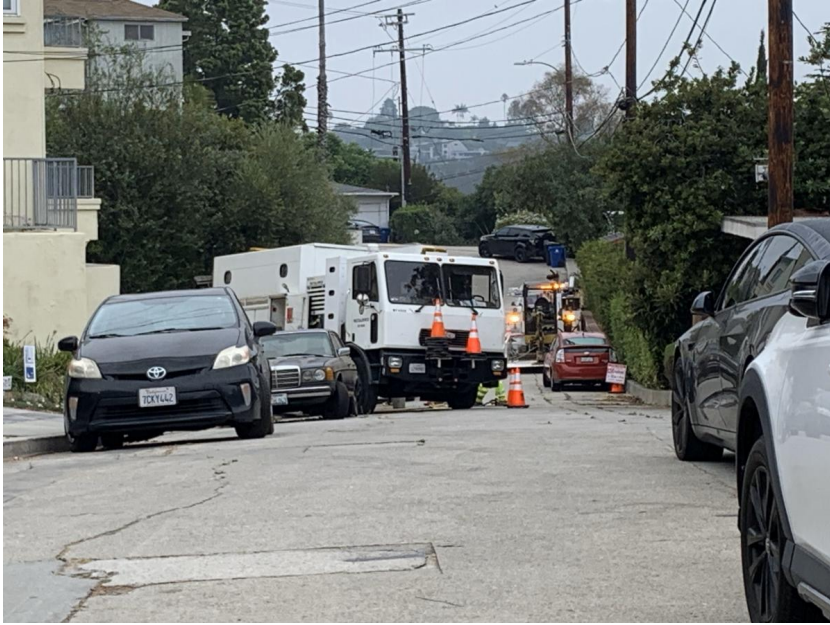
The culprit leak being repaired...
