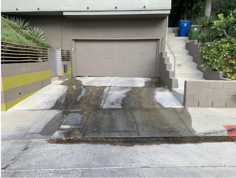
Water leaking from a home on W. Silver Lake Drive
